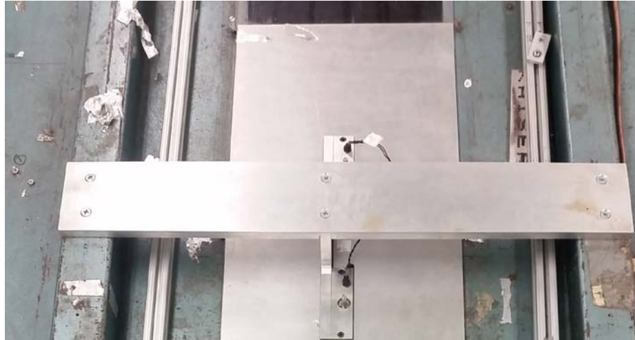
Figure 40 Model Support Top Plate Installed
